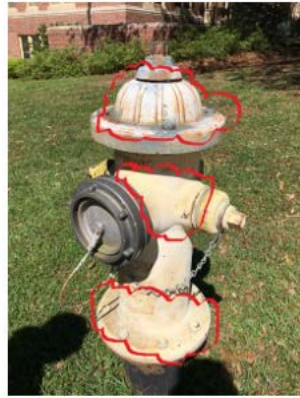
Paint is completely faded and rusted
