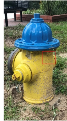
Figure 1: QR Code Placement QR code should be placed within the red outlined area.
