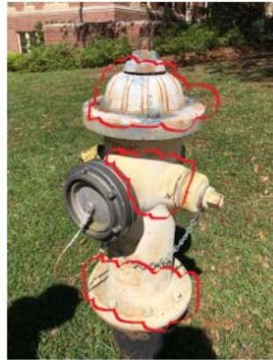
Paint is completely faded and rusted
