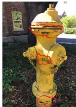
Oxidation and Cracking
