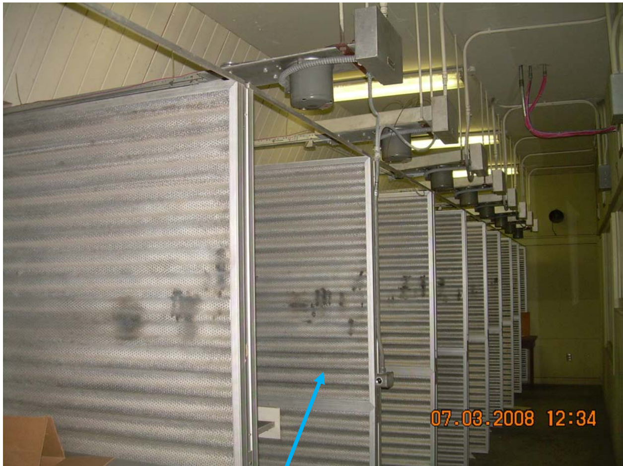
Photo 3 – Shooting Booths – Firing range, clean, remove, wrap and dispose
