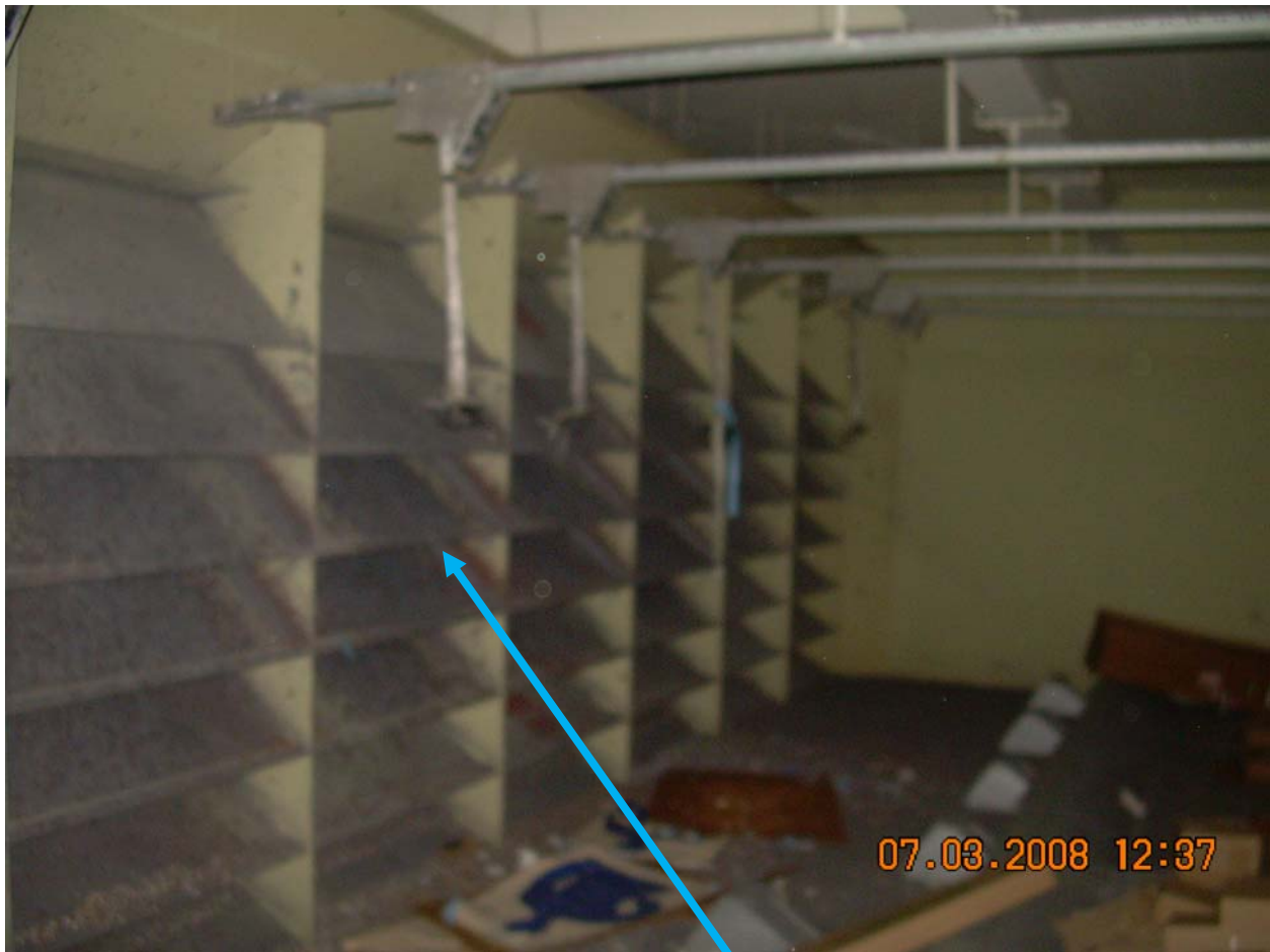
Photo 4 – Firing range – Baffles to be demolished to access back of this wall
