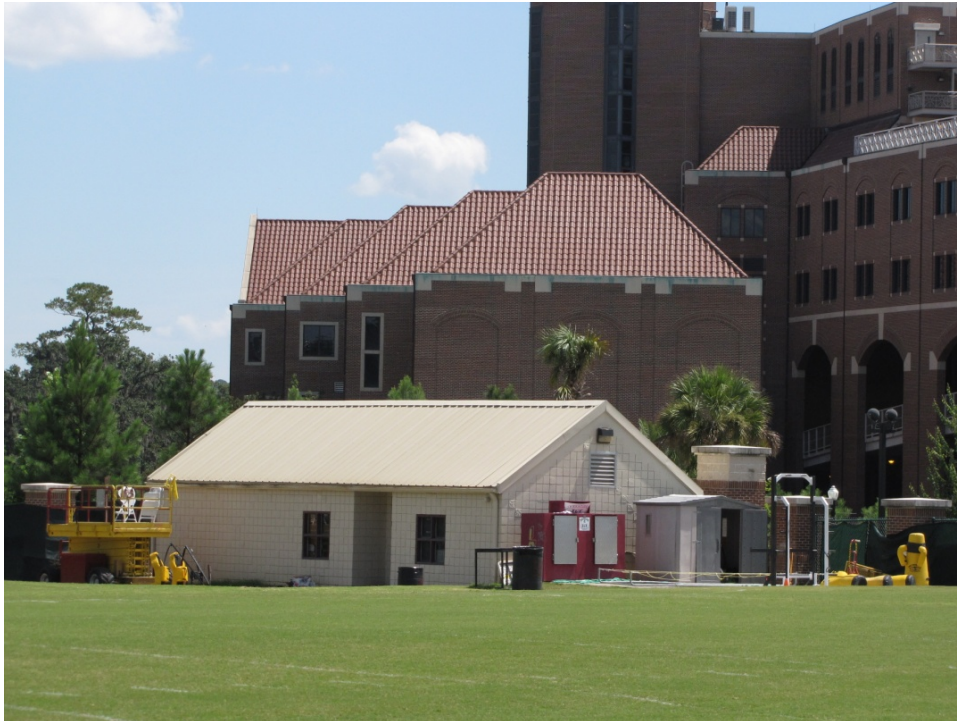
The Practice Facility Training Room (PFTR) with Ice Machine and detached storage shed outside. The building complex in the distance is the DeVoe L. Moore University Center.
