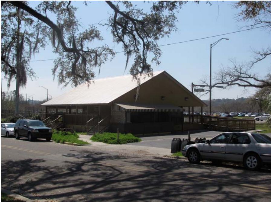
Looking toward Tribal Bar and Grill. Dunnwoody Street is in the foreground. The University Center parking lot is in the background.
