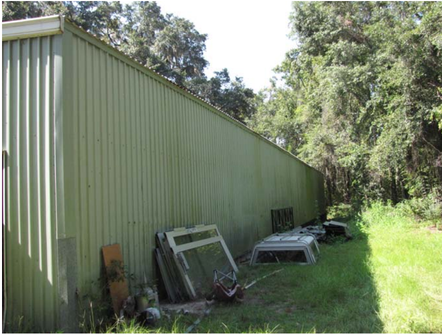
Existing metal storage shed located southwest of the proposed building site.
