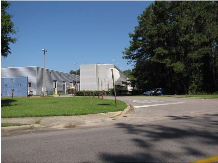
Parking and Service Entrance on E. Paul Dirac Dr., just north of Levy Avenue. Metal structure to left is the OPMD Building, structure to right contains cooling towers. Blue tile wall in foreground screens electrical equipment and service.
