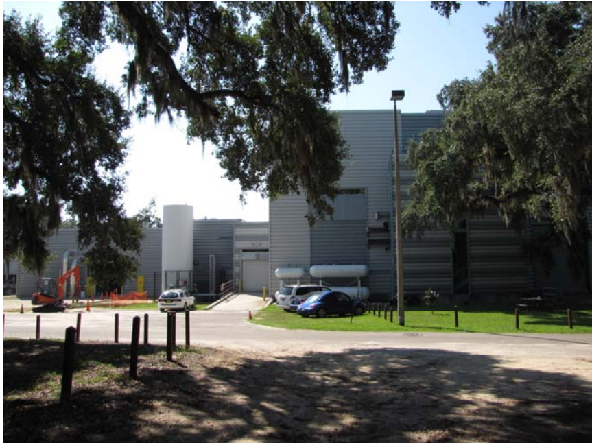
Looking southeast from the proposed site. Service drive to receiving is in the middle ground. In the background to the left are the cooling towers and to the right is the OP/MD building.
