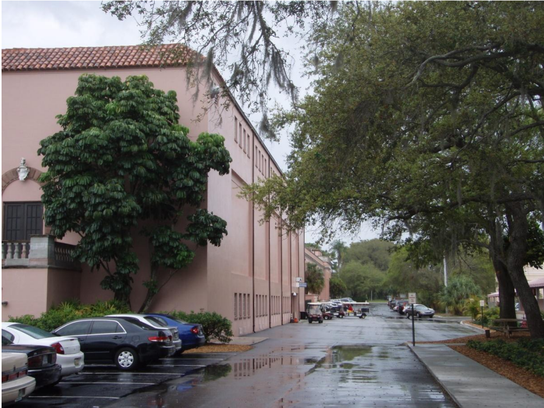
View of southwest corner of the West Wing and service drive south of the building
