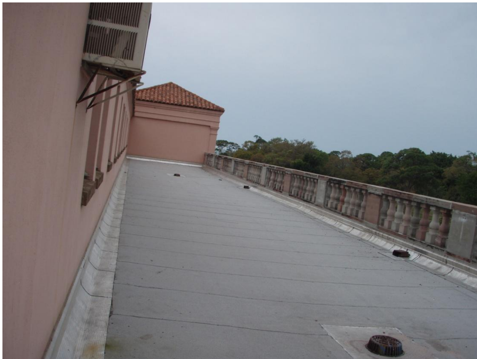
3 rd floor roof terrace
