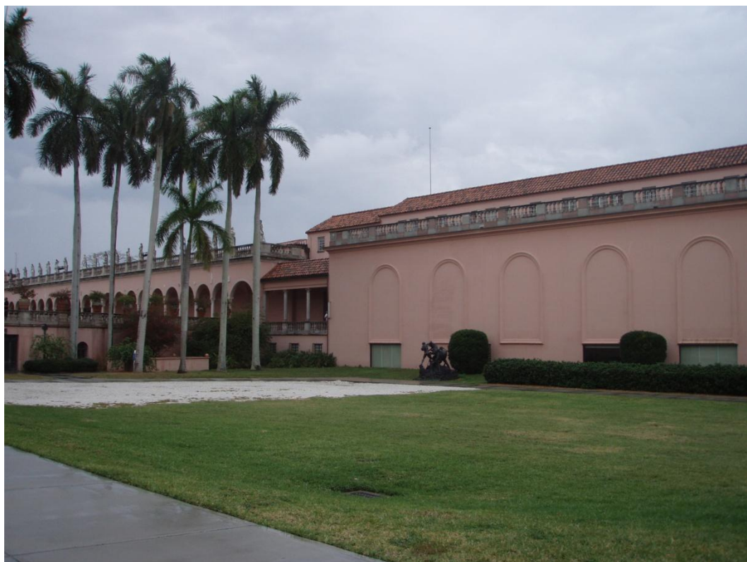
View of northeast corner of the West Wing connecting to the original arcade
