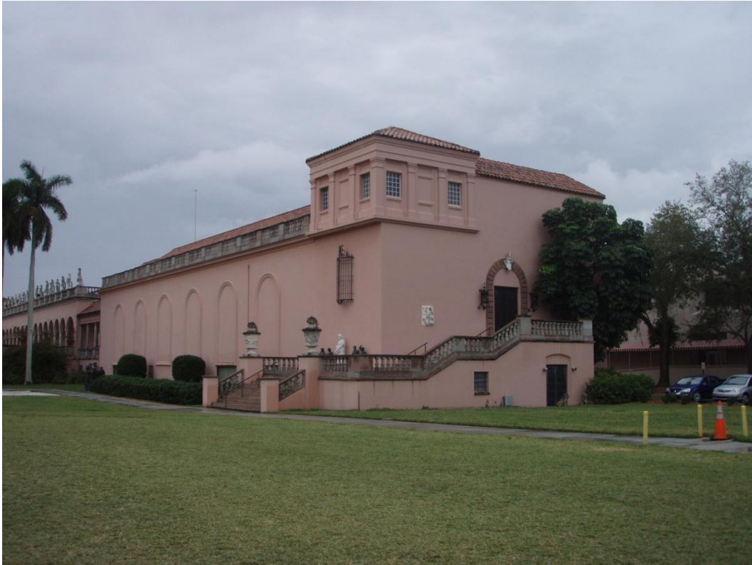
View of northwest corner of the West Wing
