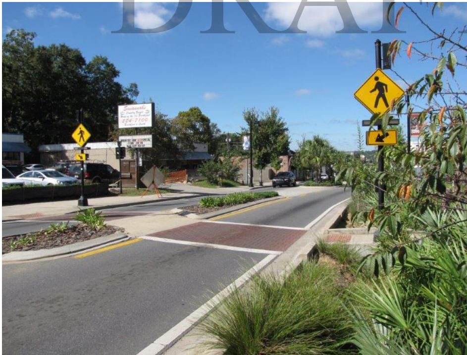
The proposed site as access to this midblock crossing. It also has a pushbutton activated beacon.
