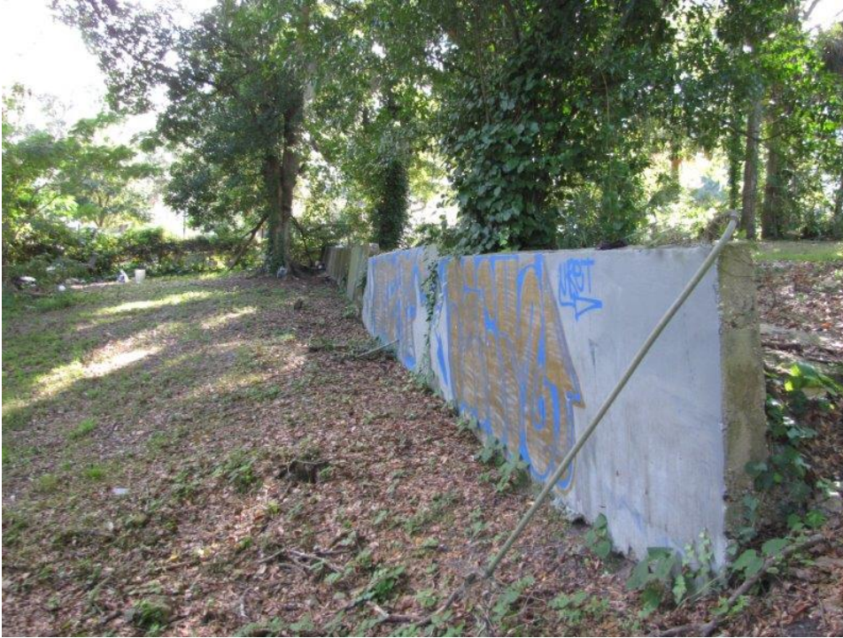
The east end of site has retaining walls, remnant of previously subdivided parcel.
