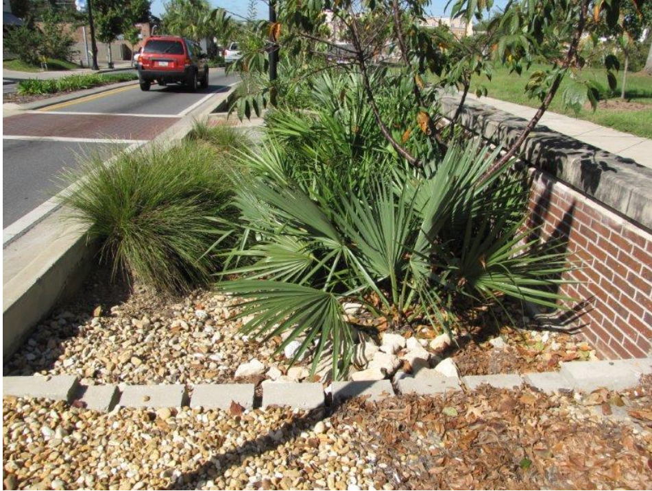
Landscape features along Gaines St. include bio-swales.
