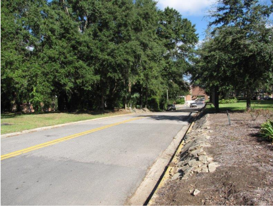
Looking north along MLK South Blvd. Site is on the left and Burnette Park is on the right. Metered parallel parking is on the west side of the street but there are no sidewalks on either side adjacent to the street. This road lines up with the east drive of the Tucker Center.
