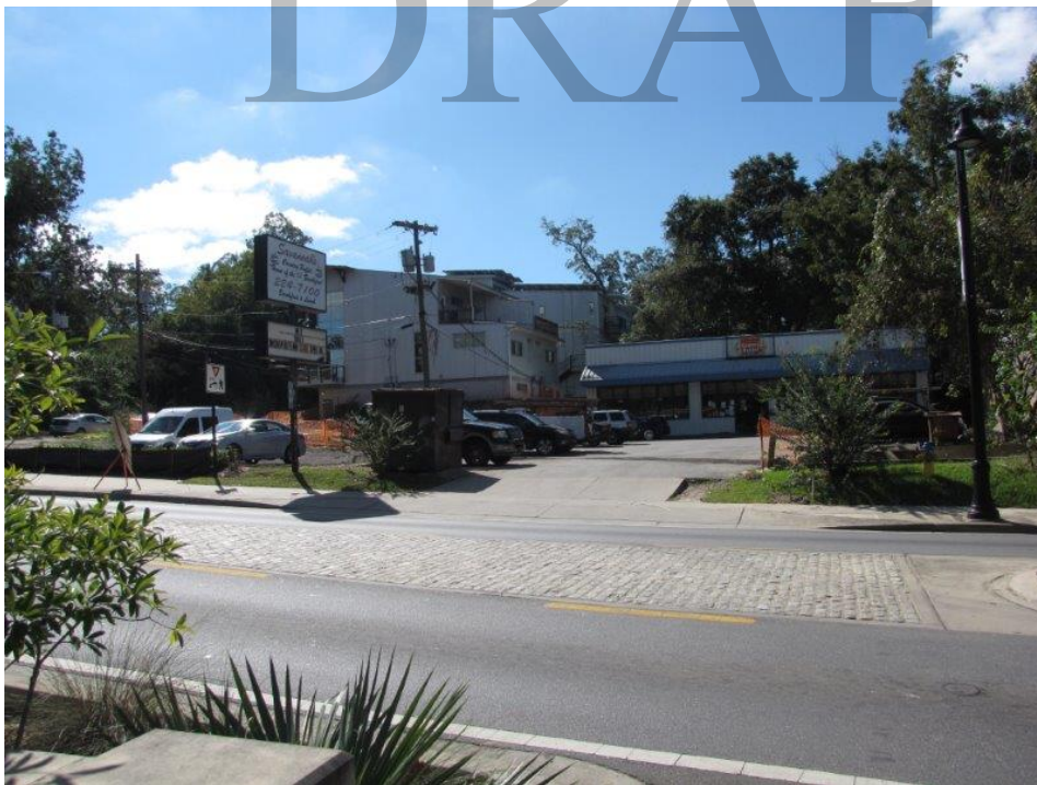
On site looking east toward retail buildings.
