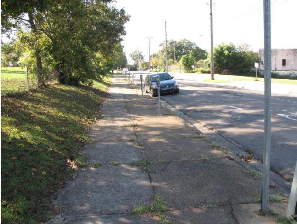
Macomb St. looking south, building site is on the left. Sidewalks are in need of minor weed control. Parallel metered parking is on the east side of the street and overhead power lines are on the west side.
